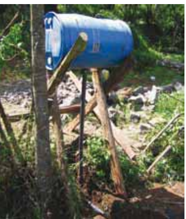
A home made water tank
