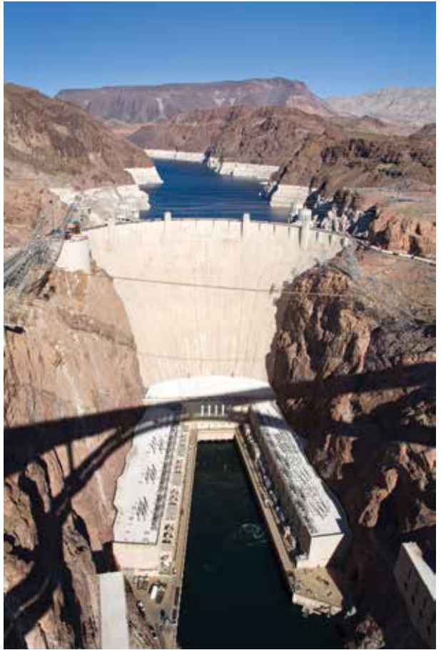
A large hydroelectric plant at the base of Hoover Dam on the Nevada/Arizona border.
