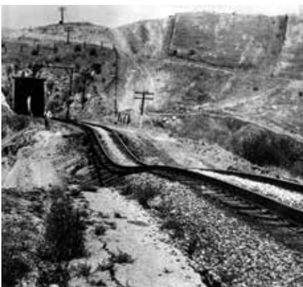
Damage caused by earthquakes
