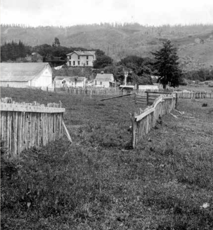
Effects of the 1906 San Francisco earthquake
