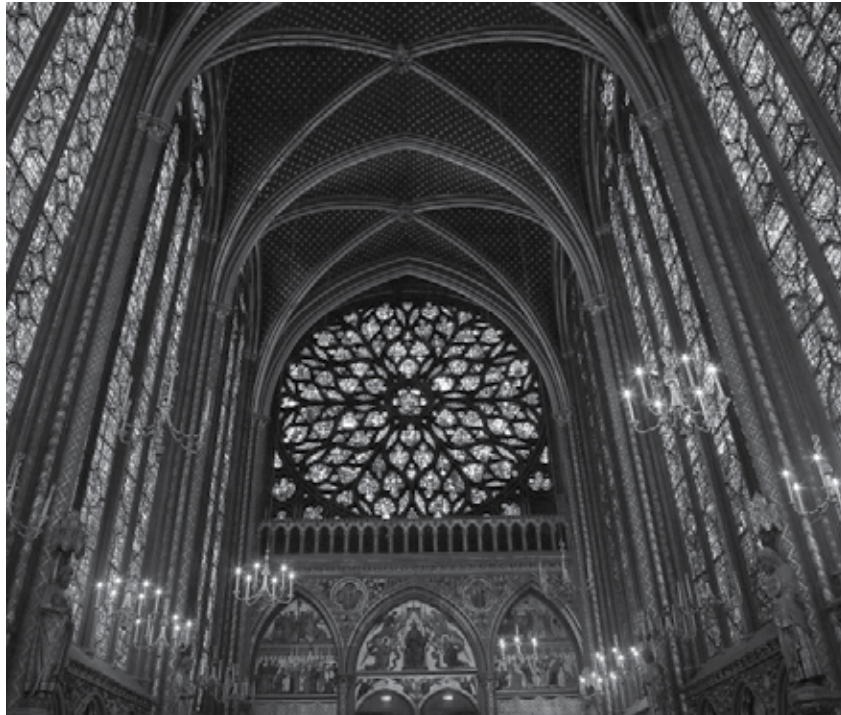
Stained-glass windows in La Sainte-Chapelle in Paris, France, built in the 1200s
