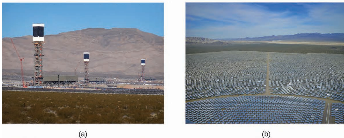
Figure 5.10 (a) The Ivanpah solar thermal plant uses 170,000 mirrors to concentrate sunlight on water-filled towers. (b) It covers 4000 acres of public land near the Mojave Desert and the California-Nevada border. (credit a: modification of work by Craig Dietrich; credit b: modification of work by "USFWS Pacific Southwest Region"/Flickr)
