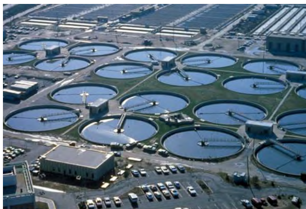
Figure 15.6 Wastewater treatment facilities, such as this one, remove contaminants from wastewater before the water is released back into the natural environment. (credit: "eutrophication&hypoxia"/Wikimedia Commons)
