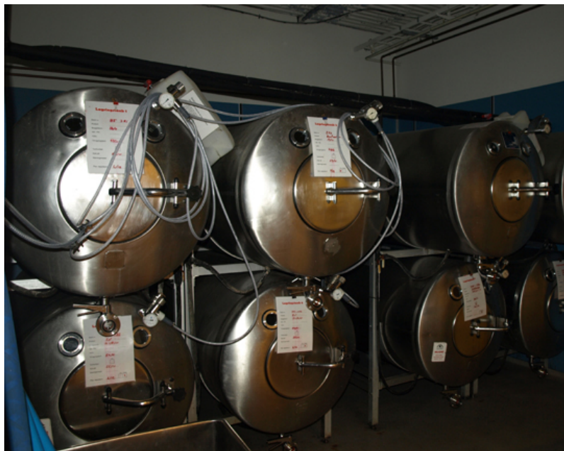
Figure 6.13: Fermentation of grape juice to make wine produces \text{CO}_2 as a byproduct. Fermentation tanks have valves so that pressure inside the tanks can be released.
