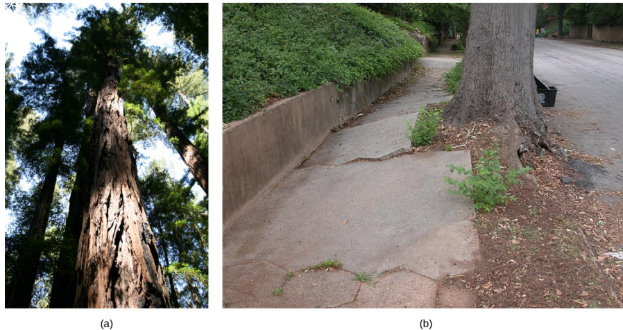
Figure 23.18 With heights nearing 116 meters, (a) coast redwoods ( Sequoia sempervirens ) are the tallest trees in the world. Plant roots can easily generate enough force to (b) buckle and break concrete sidewalks, much to the dismay of homeowners and city maintenance departments. (credit a: modification of work by Bernt Rostad; credit b: modification of work by Pedestrians Educating Drivers on Safety, Inc.)
