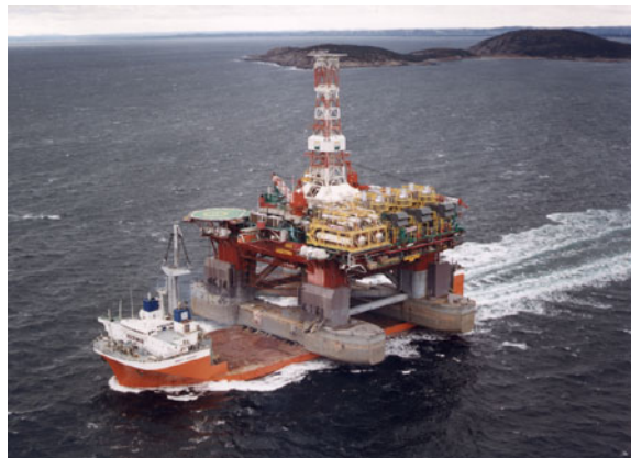
Figure 7.4: The Petrobras P-36 oil platform.
